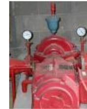
Current regulations require a towing vessel to be equipped with a self-priming fire pump; which may be either fixed or portable. Owners whose vessels have fixed pumps should ensure that the pump has been fitted with a remote start control and that the control is in working order.
